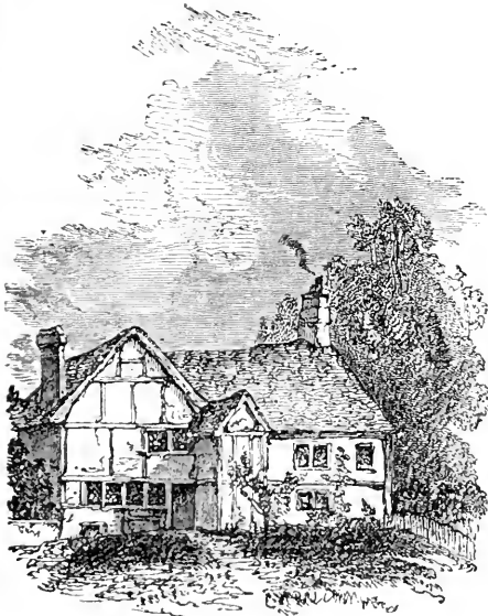
Milton's Cottage at Chalfont.
